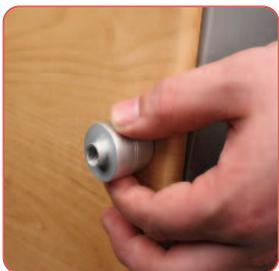
Replace the top set of turn parts on the front of the counter with the stand off kit
